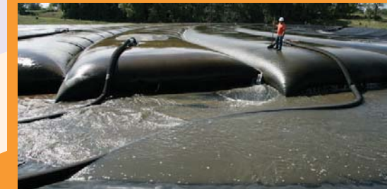
Silt separation with Geotube
