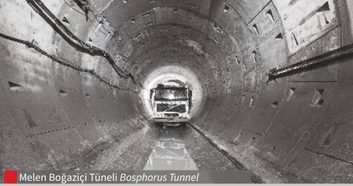
Melen Boğaziçi Tüneli Bosphorus Tunnel
